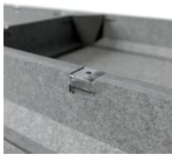
Box Tile Double Beams Clip Detail
